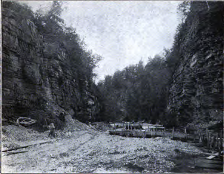
FIG. 1.—SITE OF SIX-MILE CREEK DAM.
